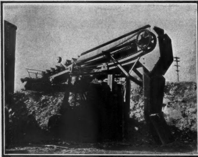
Link-Belt Loader and Buda Engine in Operation
